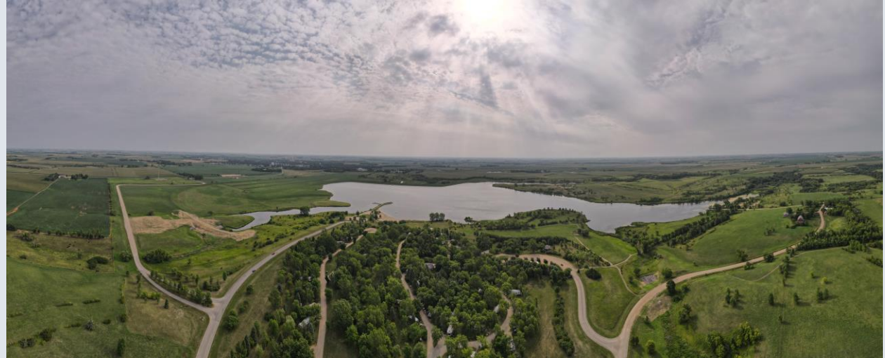
Aerial photograph of a capital projects implemented by the project partners to protect and improve Del Clark Lake. On the left, there are two grade stabilization structures. On the right, one road retention project.
